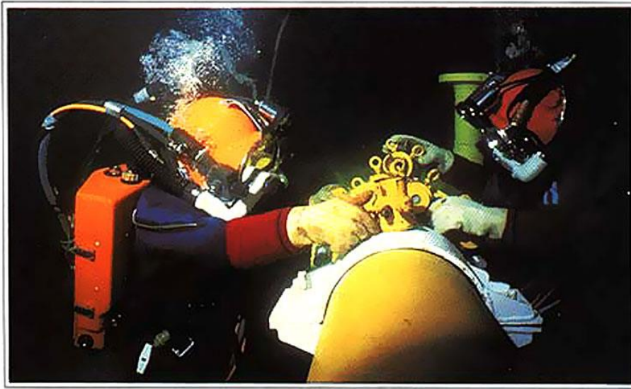
DIVERS CONNECTING A PIPELINE AT A DEPTH OF 520 METRES.
