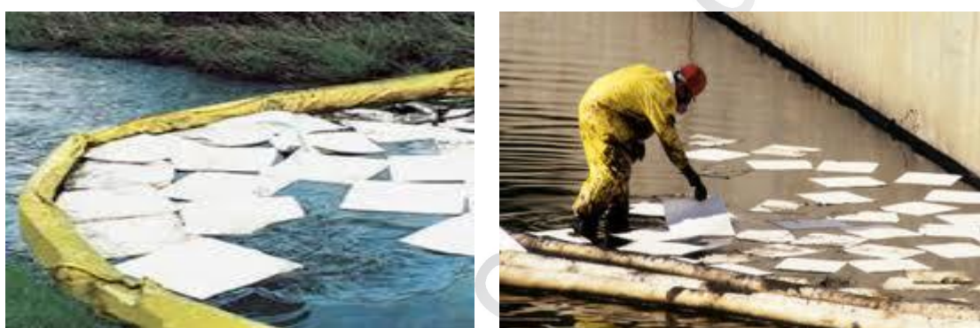
Fig. 1.18 Use of adsorbents at sea (left), in the port (right), [OSS]
