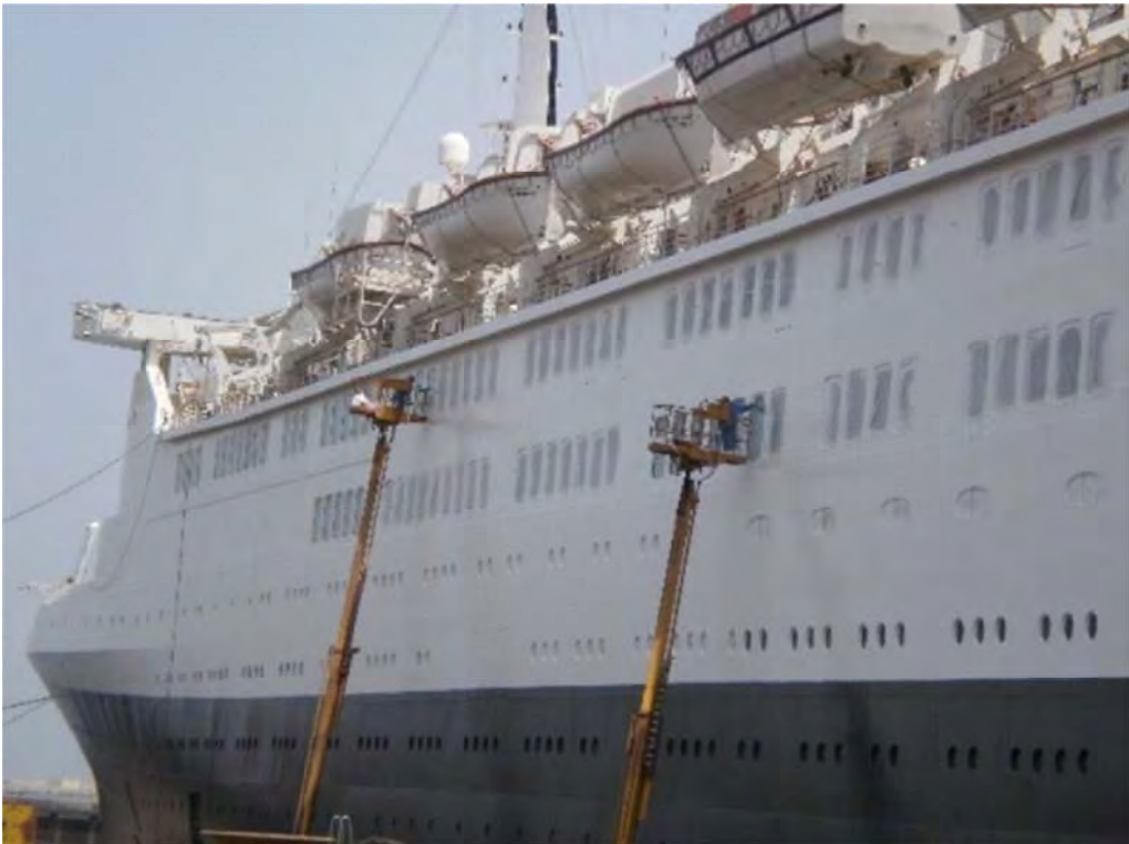
Picture 18: Superstructure painting
