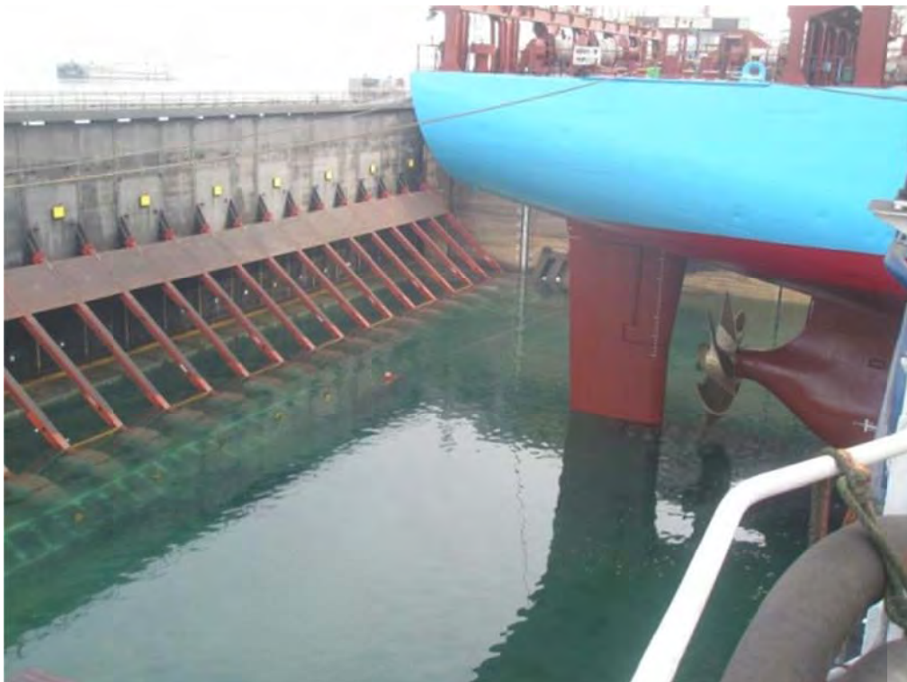
Picture 4: Graving dock is drying
