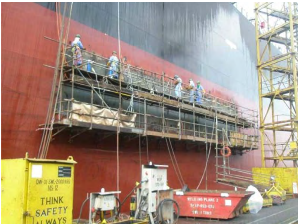
Picture 20: Side shell steel repair
