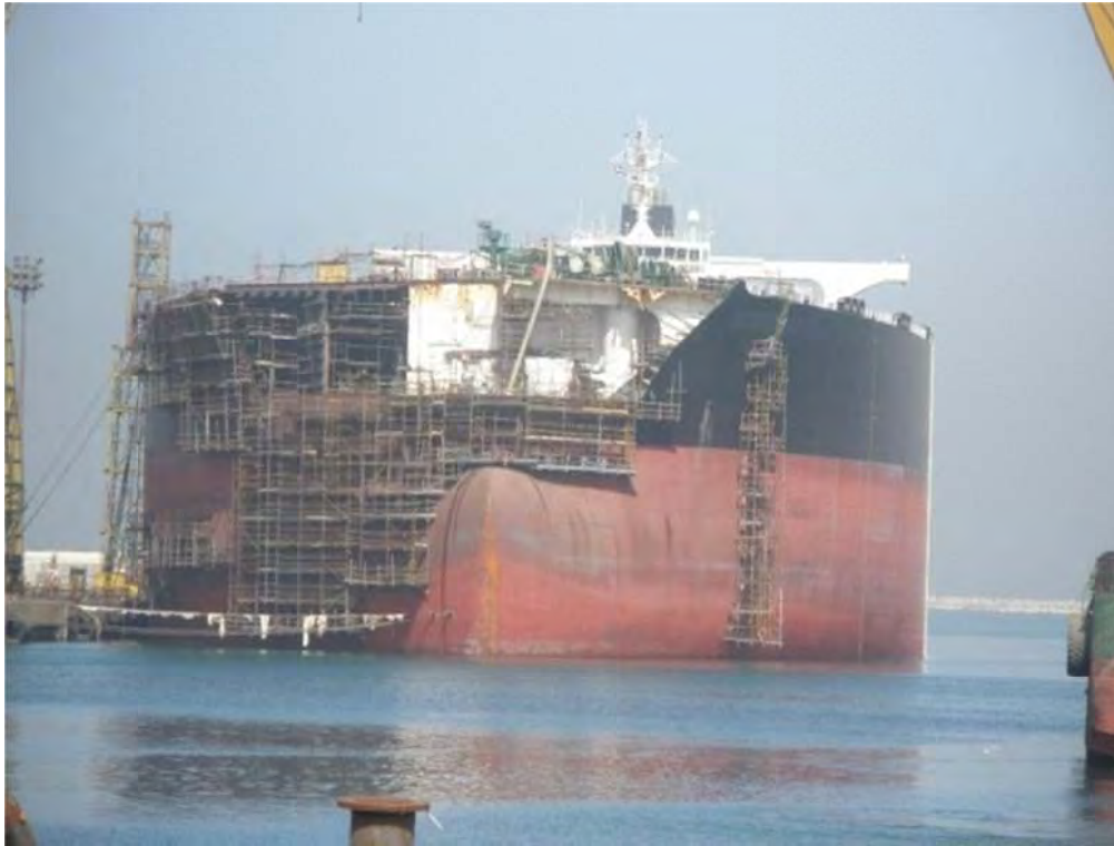
Picture 27: Afloat steel repair after collision
