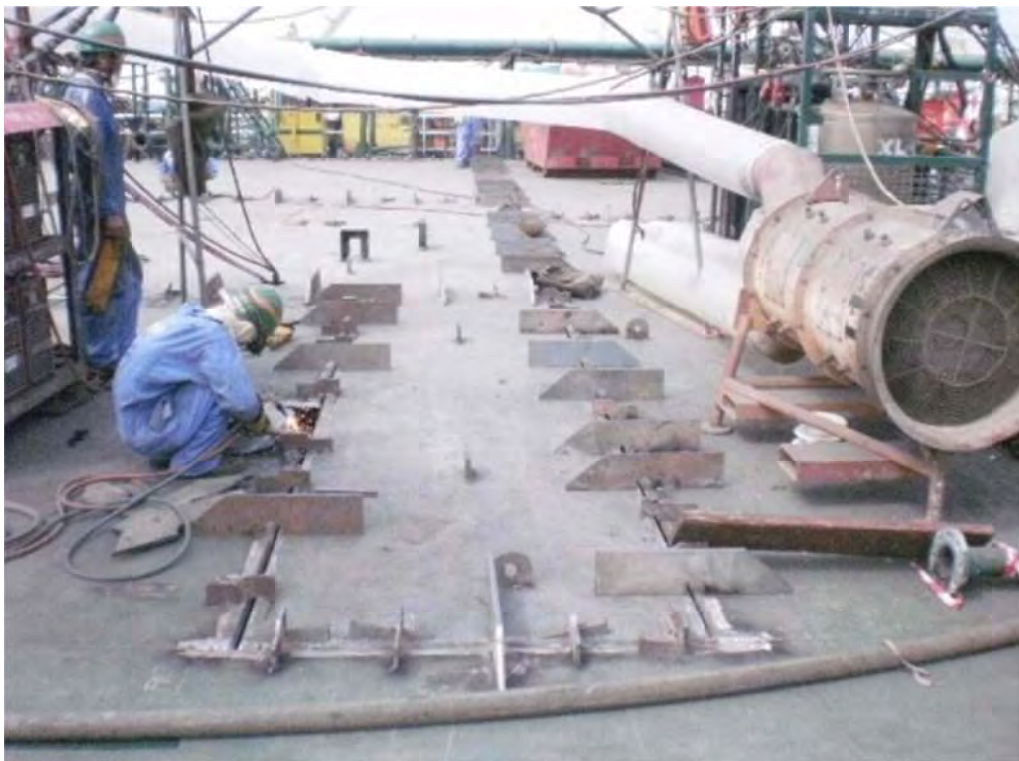
Picture 24: Main deck steel plate repair
