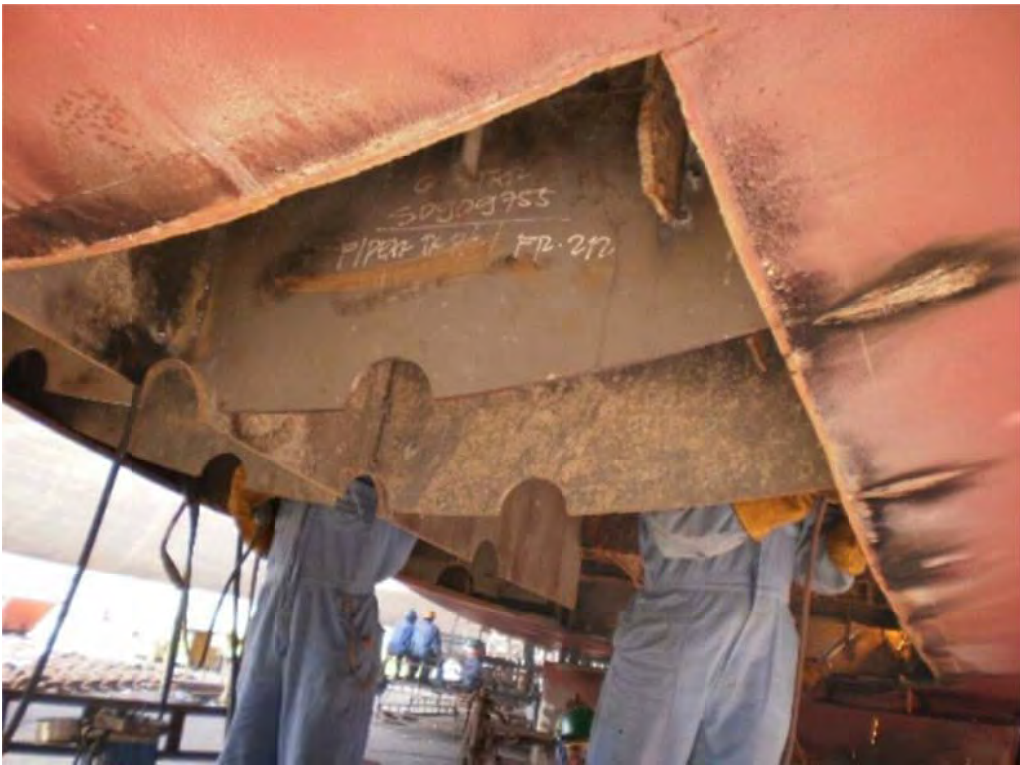
Picture 22: Bottom shell steel repair
