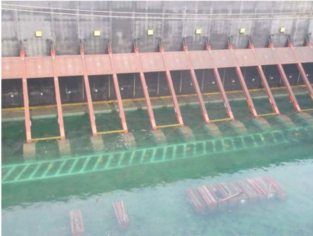
Picture 3: Graving dock is drying
