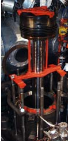
(Photo No 4, Overhauling of Piston Crown at Vessel M/V SEABOSS, Ref.[17])
