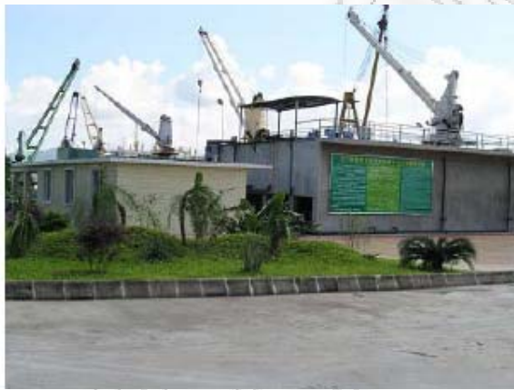
Figure: The waste water treatment center at Zhongxin's Xinhui yard, Source: Present Situation and Future Development of the Ship Recycling Industry in China, Mr. Xie Dehua Executive vice-chairman & Secretary-general of China National Shiprecycling Association, June 6, 2007 Hong Kong, China
