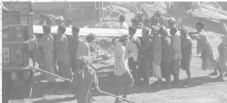
Figure: Loading of metal plate on truck, Source: Ship Breaking Activities and its Impact on the Coastal Zone of Chittagong, Bangladesh: Towards Sustainable Management , Young Power in Social Action (YPSA), July 2006
