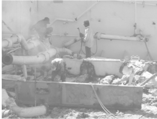
Figure: Workers take out asbestos and glass wool from engine room of scrapped ship without having any protective tools, Source: Ship Breaking Activities and its Impact on the Coastal Zone of Chittagong, Bangladesh: Towards Sustainable Management , Young Power in Social Action (YPSA), July 2006
