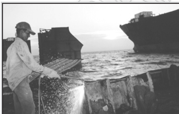
Photograph 3 : A labour of cutter group is cutting iron plate.
