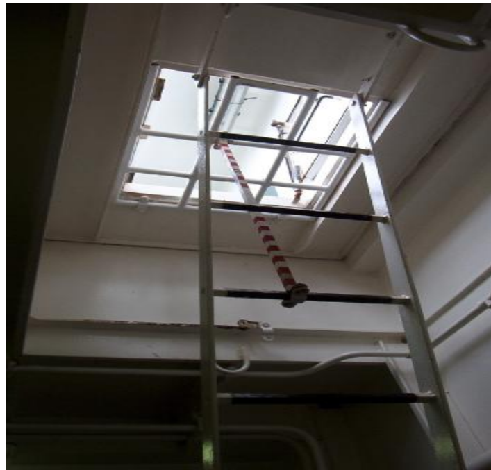
Exit grate bars permanently closed
