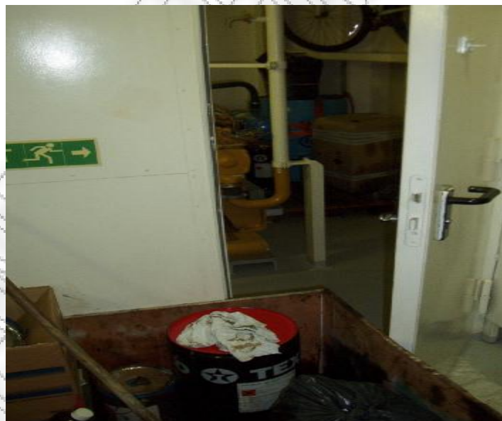
Emergency door blocked
