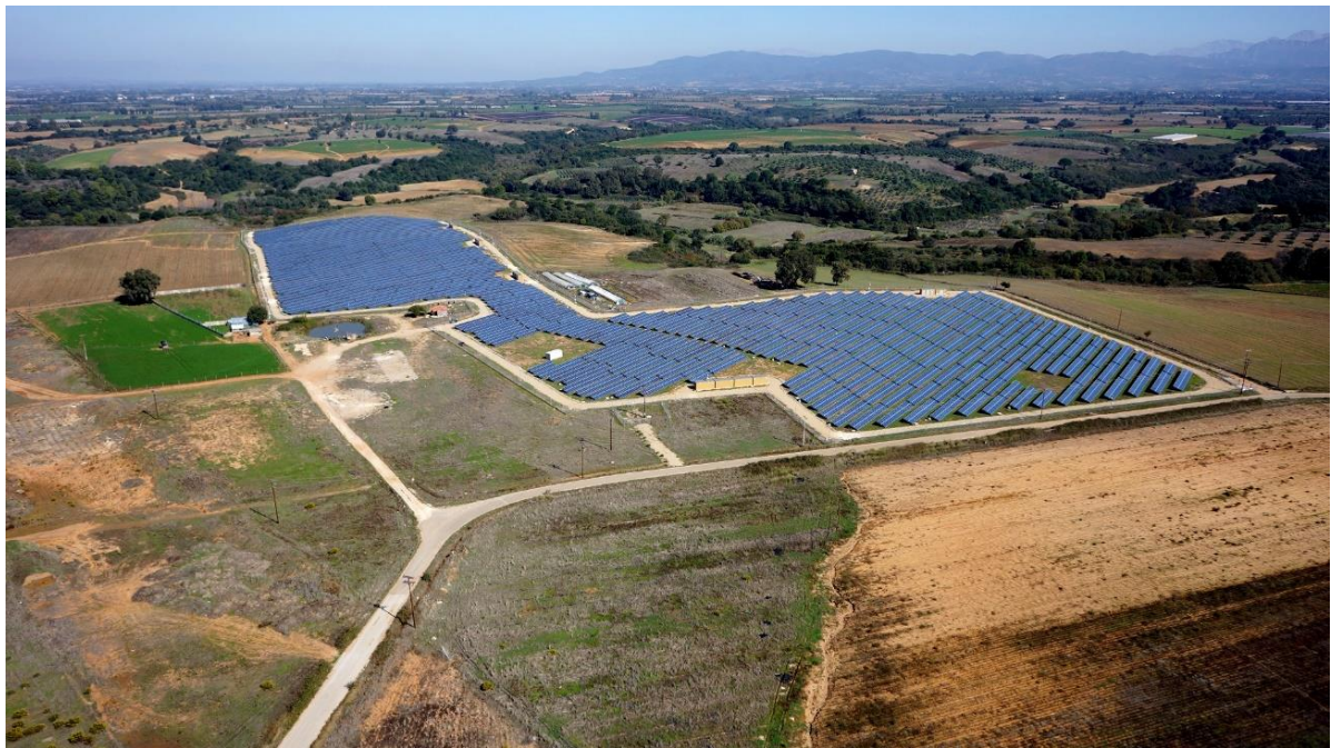
Picture 1. The photovoltaic park of Kourtesi from above.
