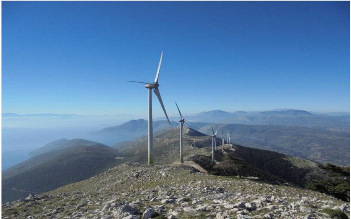
Picture 3. View of Panachaiko wind park.
