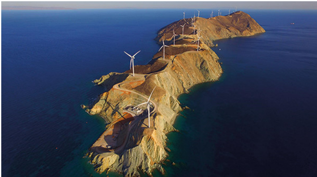
Figure 8: The onshore wind farm, with offshore characteristics, in the island, Saint Georgios, in Greece
