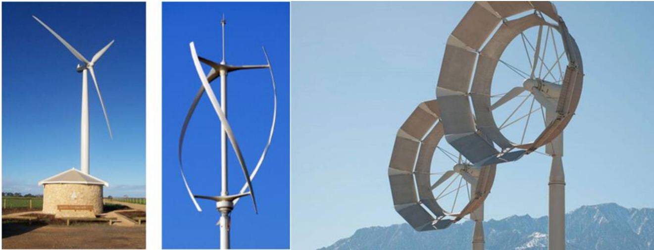
Figure 6. Examples of HAWTs (left), VAWTs (middle) and Shrouded HAWTs (right). Sources: https://quintongraybealsanmarin.weebly.com/outdoor-classroom-design.html & http://www.wind-works.org/cms/index.php?id=541
