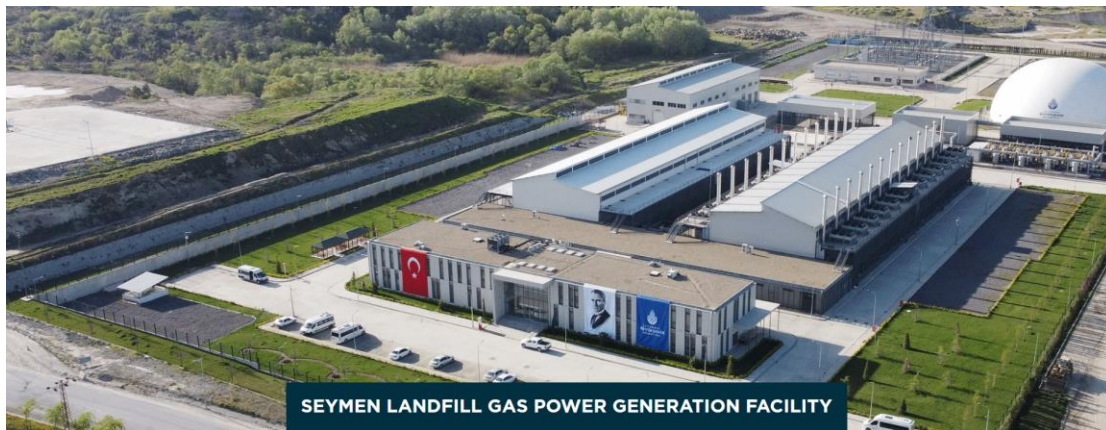
Figure 15: The Seymen landfill gas power station. It may be the beginning of the utility of biomass, (Source: BMF Enerji)
