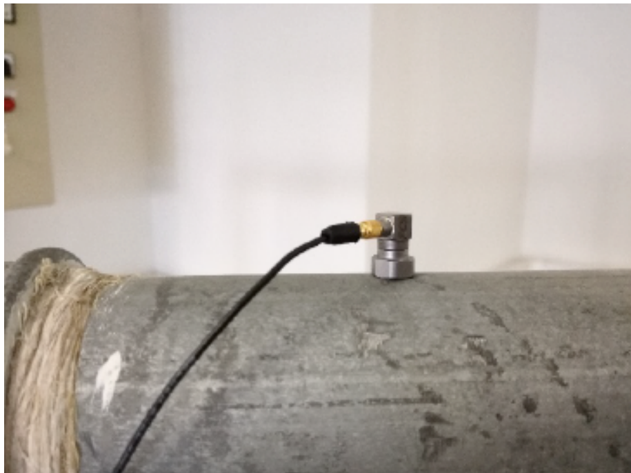
Figure 64. Mounting a vibration meter on a network section [11-13]
