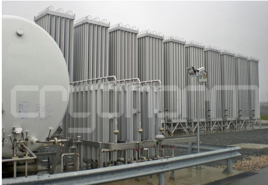
Figure 5. Ambient air vaporizer (Source: Cryonorm.com)
