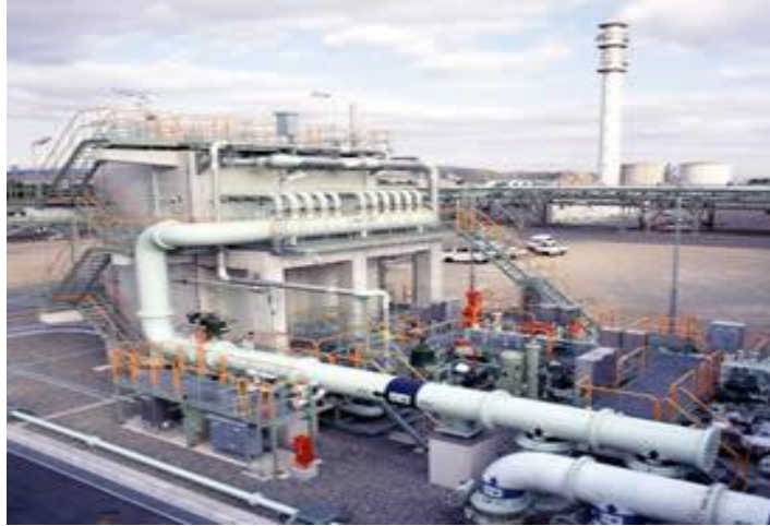
Figure 3. Open Rack Vaporizer (Source. Kobe & Steel LTD)
