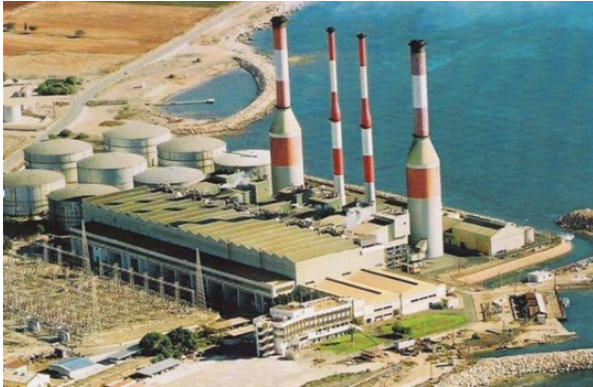
Photo 2.1: Aerial photo of Dekelia Powerplant [1-14].
