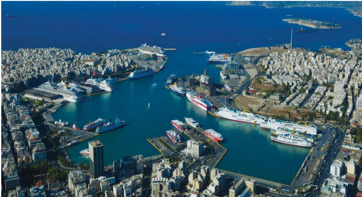
Figure 9 Ferry terminal of Piraeus Port, Piraeus Port Authority S.A, 2018, https://www.olp.gr , Access on 29 March,2022
