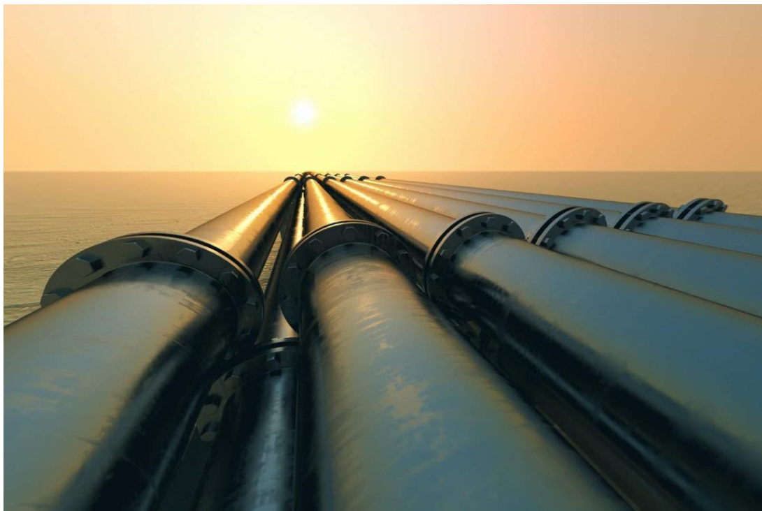
Image: A pipeline project. Photo: courtesy of outgunned21/Freeimages.com.
