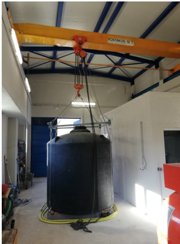
Crane bridge and water tank for lifting, for its certification
