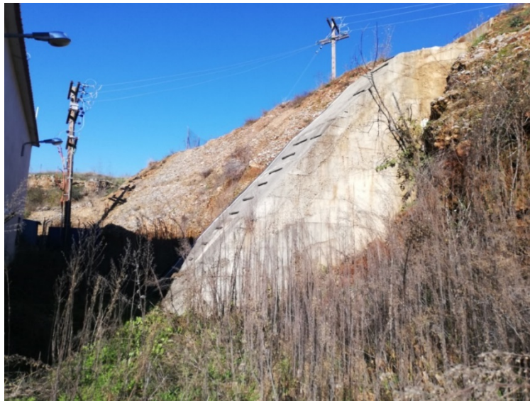
Concreted penstock
