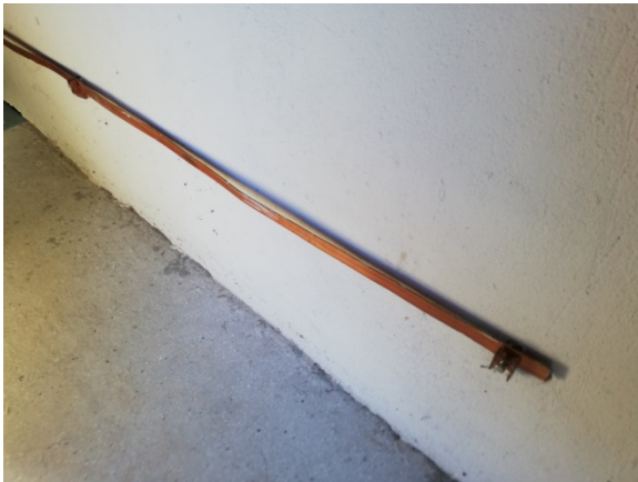
Grounding copper bars at the M.V. cubicles and the L.V. panels
