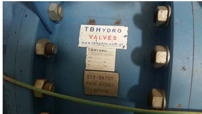
Main Inlet Valve label
