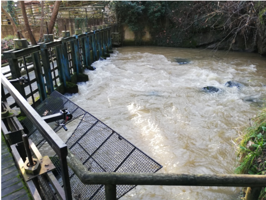
Water intake and protection mesh at the springs of Enipeas
