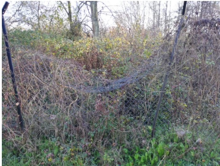
Fencing of the power house
