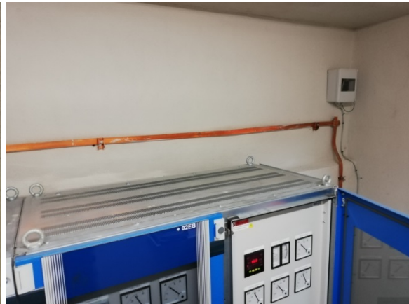
Grounding copper bars at the M.V. cubicles and the L.V. panels
