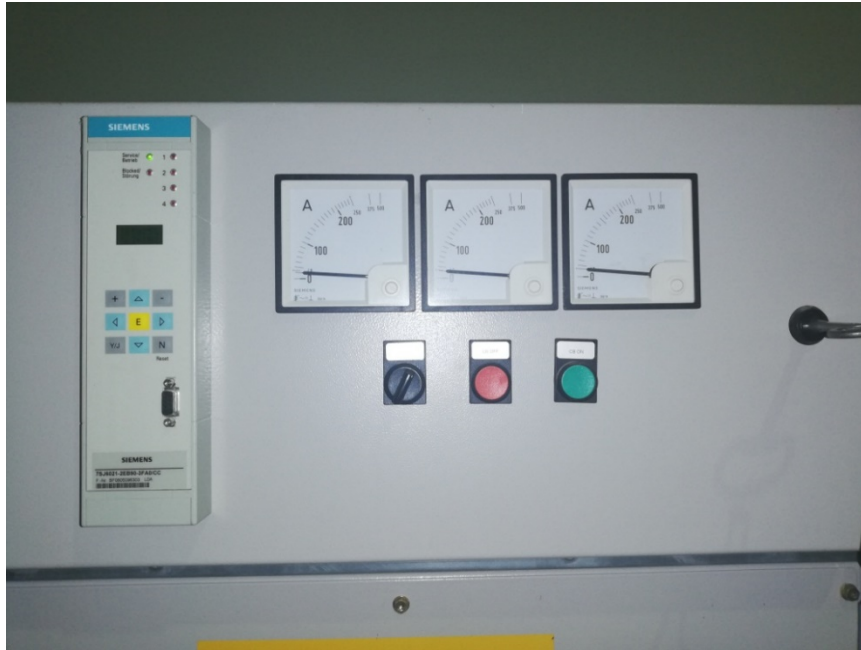
Medium Voltage Protection Relay
