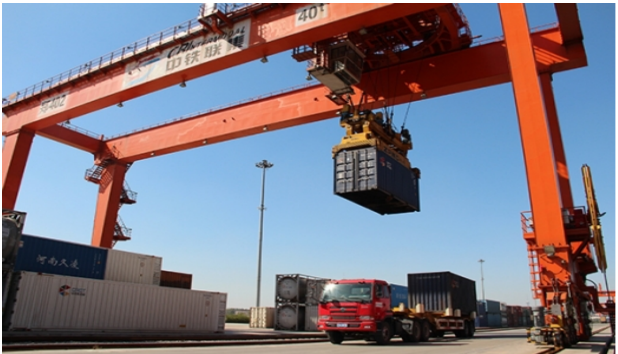
4. Yard Gantry Crane
