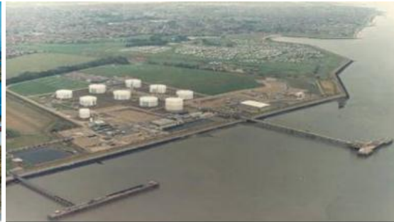
Canvey Island Receiving Terminal, UK
