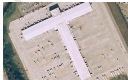
T-shaped crossdock in Atlanta, GA (American Freightways)
