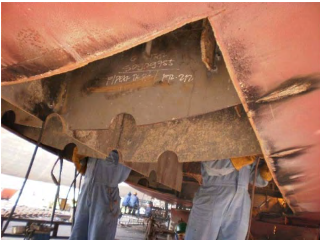
Picture 22: Bottom shell steel repair
