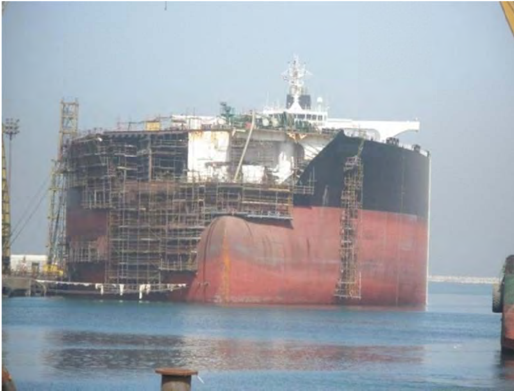
Picture 27: Afloat steel repair after collision
