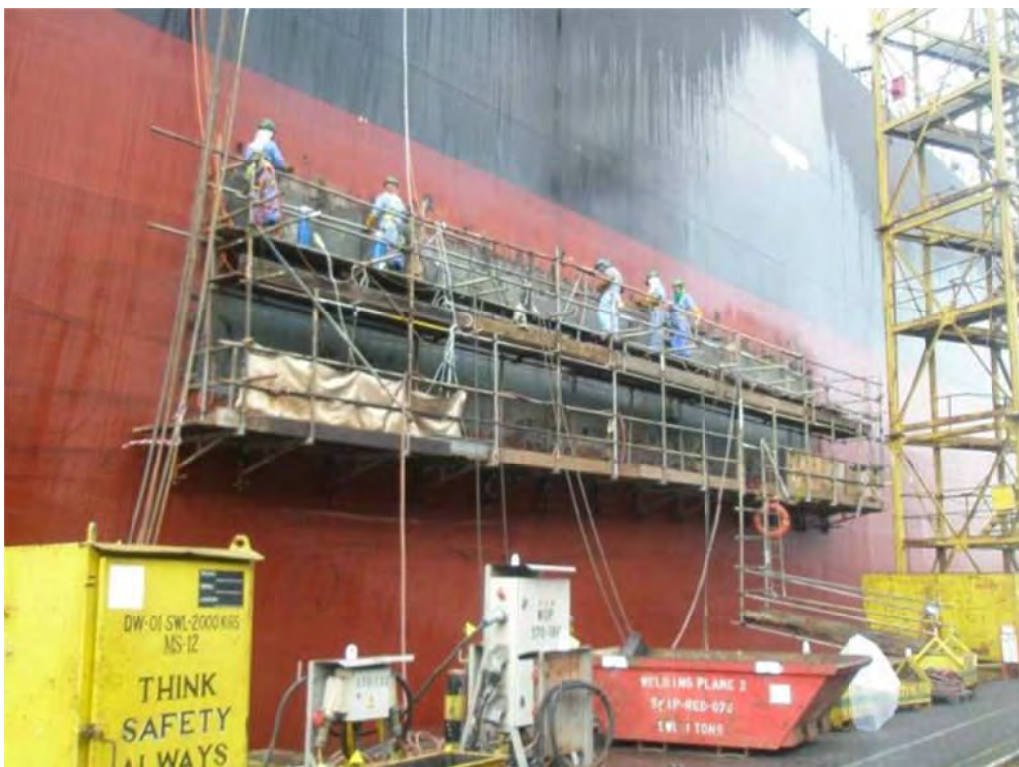
Picture 20: Side shell steel repair
