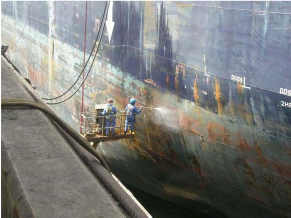
Picture 15: Side shell high pressure washing
