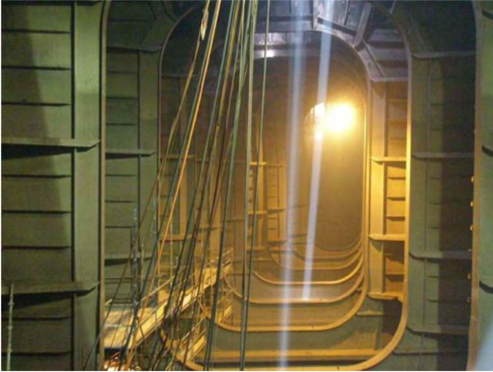
Picture 25: Steel repair in a VLCC ballast tank
