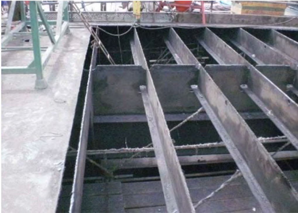
Picture 23: Main deck steel plate repair
