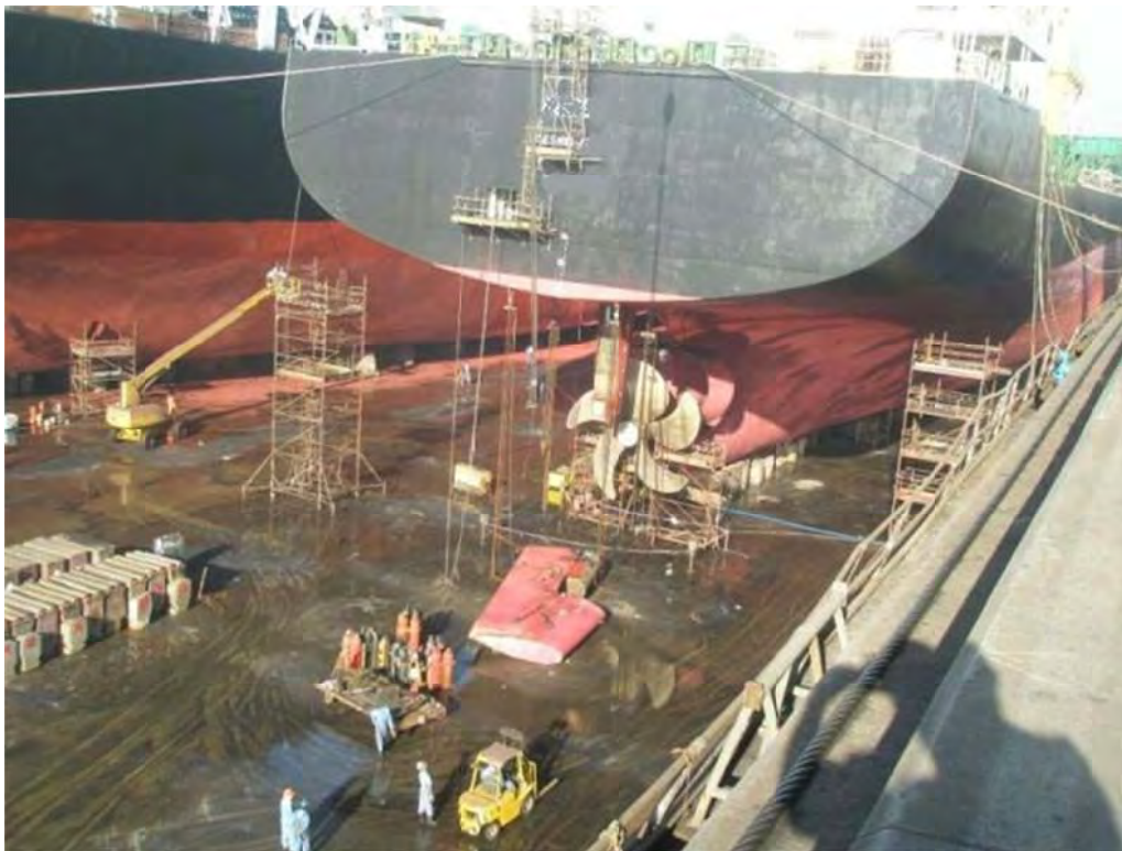
Picture 12: Rudder removal in a dry-dock
