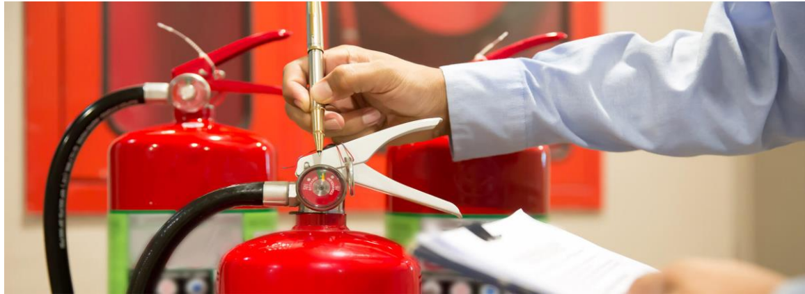
Figure 20: Fire extinguishers survey (Triton Group, 2021)
