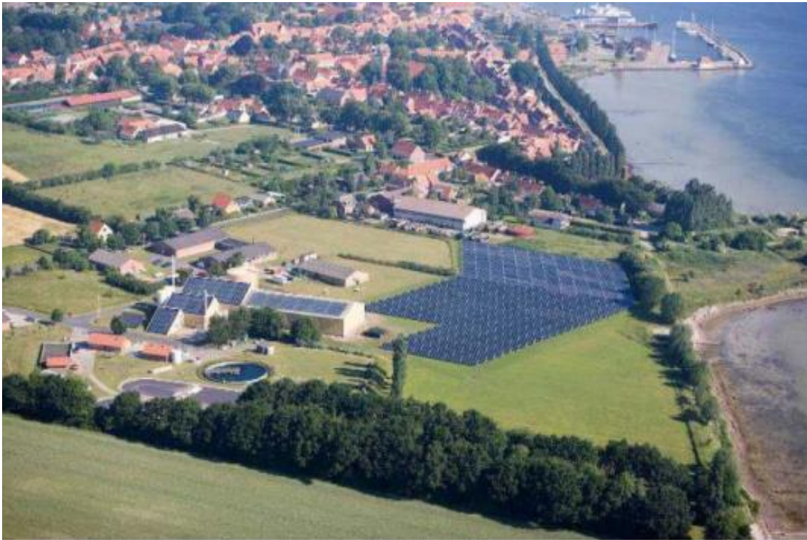
Picture 2 - Solar district heating plant in Ærøskøbing
