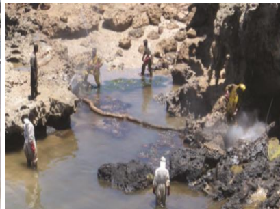
Polypropylene sorbent boom used to collect oil released during flushing operations
