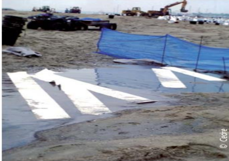
Use of Sorbents for Spill Response
