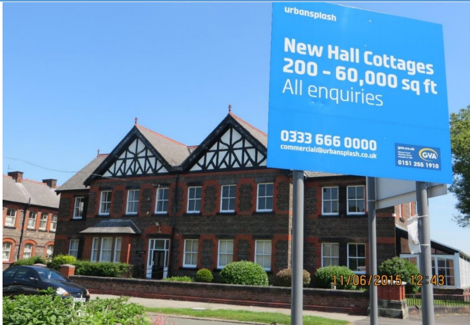
Figure 18: New Hall Cottages
