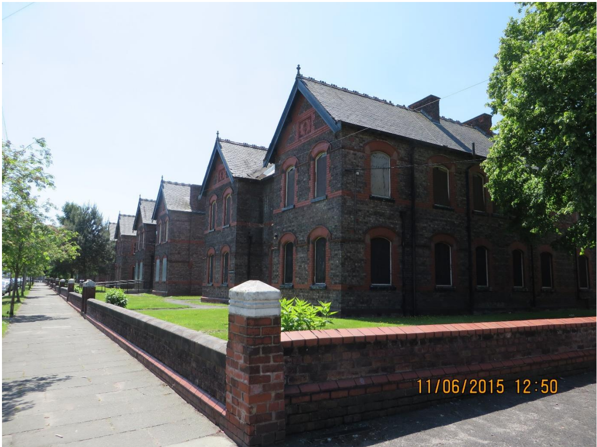
Figure 24: The front view of the Cottages
