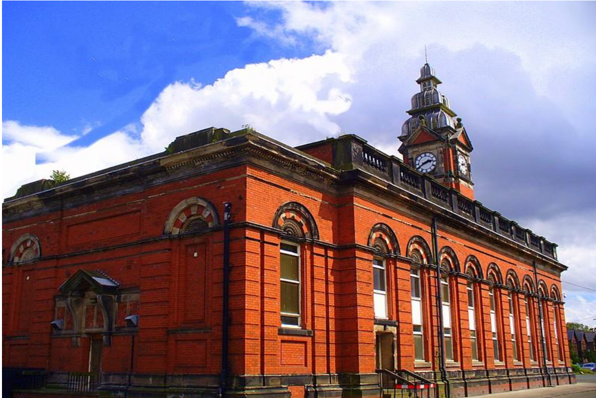
Figure 20: A back view of the tower
