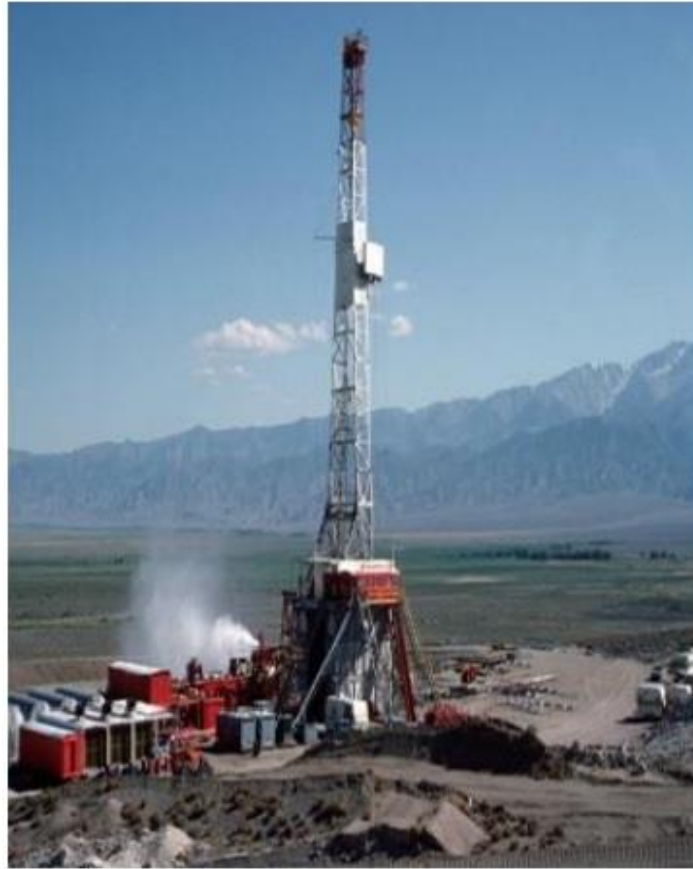
Figure 2: Drilling rig ( DiPippo, Ronald, 2012 )
